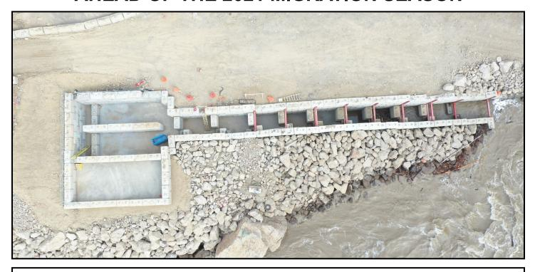
**TOP:** An aerial image of the concrete fish ladder; fish will swim up the ladder and into the holding area before being loaded into transport tanks for release upstream.
