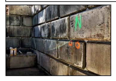
With the onset of the spring freshet, work is focused on the concrete fish ladder at the West Beach area of the site. Originally built last year, the structure is undergoing some significant upgrades. This past week crews completed the final placement of blocks to expand the ladder. They sealed and backfilled the blocks and poured the concrete base in the sedimentation basin. Handrails, wooden platforms and steel walkways are now being installed.
